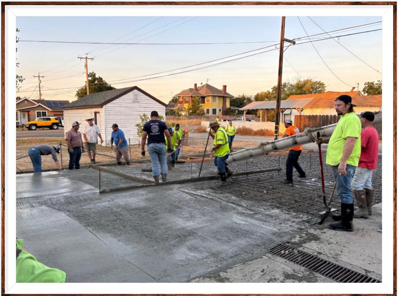
Concrete Driveway Apron Installation
