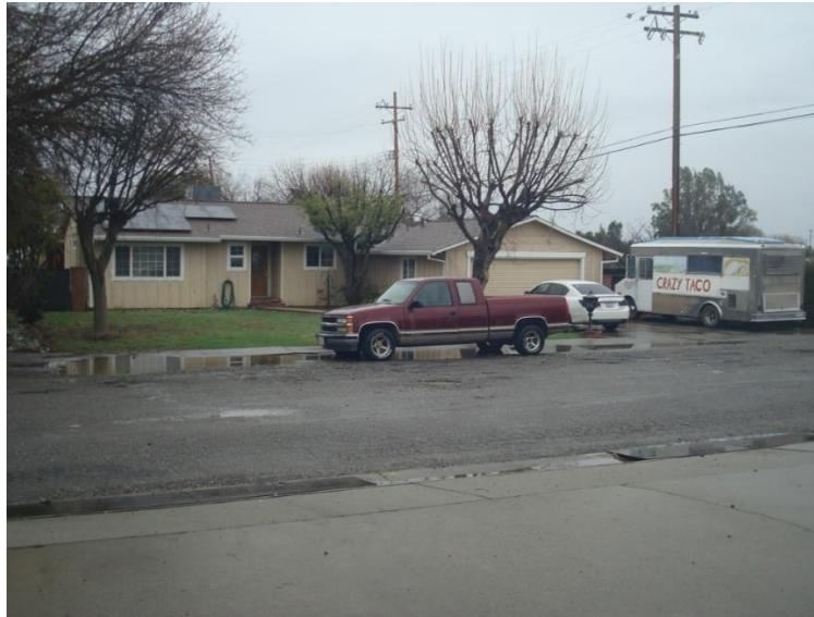
Photo 1. Every time there is much rain, there is a large puddle of water covering the sidewalk and gutter at 445 Green Street that lasts for days. This water makes it difficult for the residents to access their vehicle. Green Street repair needs to raise the lower section of sidewalk and increase slope of the gutter to drain into the field.
