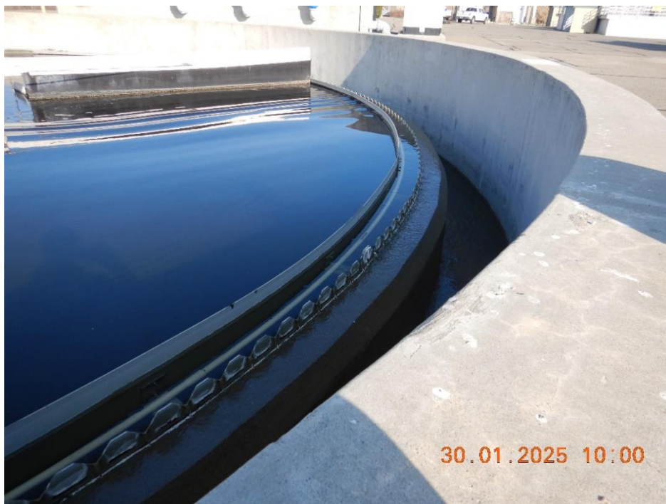
Photo 3: Effluent from Secondary Clarifier No. 1 appeared clear and free of debris.
