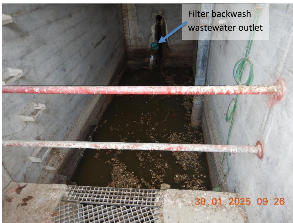
Photo 2: Filter backwash wastewater is routed back to the headworks.
