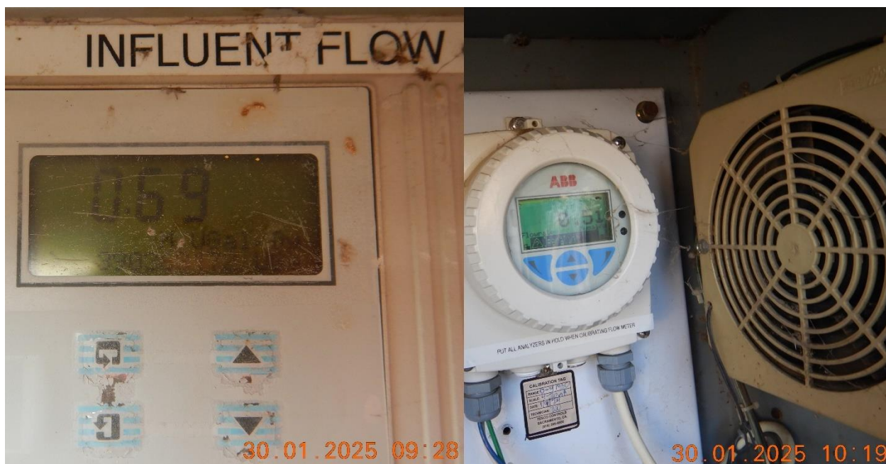
Photo 8: Influent flow meter on left showing 0.69 MGD, and effluent flow meter on right showing 0.51 MGD.
