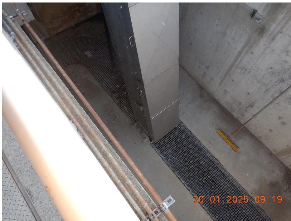
Photo 1: Newly installed automated fine screens.
